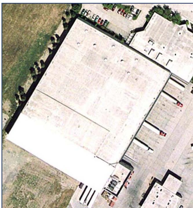
Aerial View of Project Site near Sacramento, California
